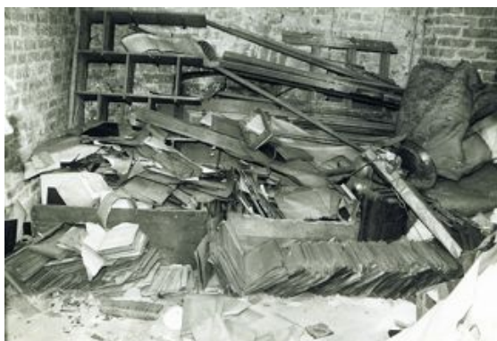
Just part of the collapsed shelving in the Sutton Shop basement
