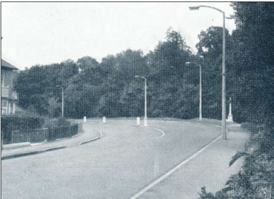
London Road, Ewell – A recent road improvement
