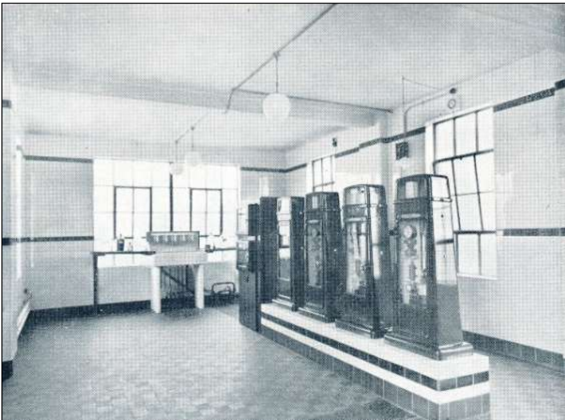
The Corporation's Water-Treatment House
